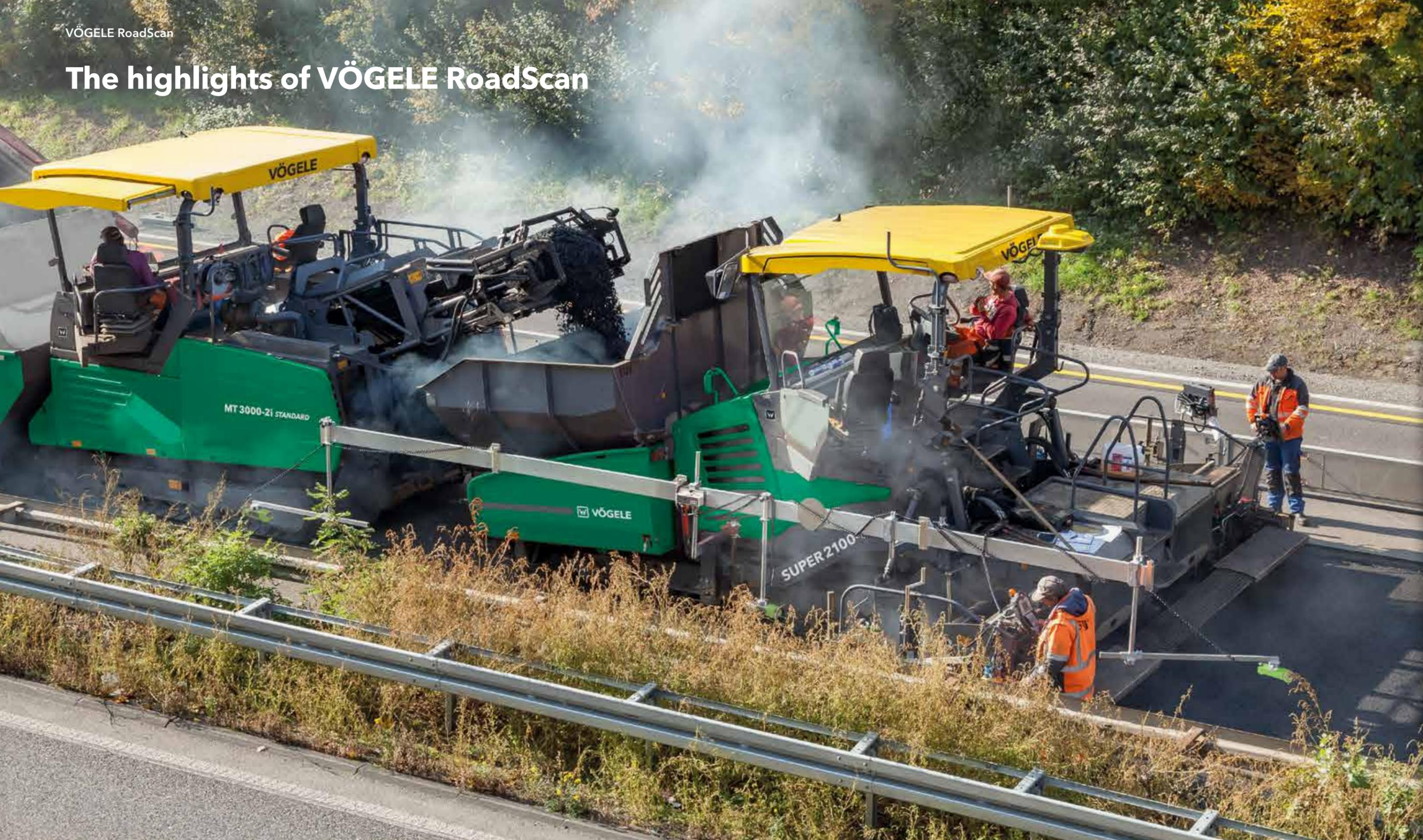
**Area-wide temperature measurement** across the entire pave width up to 10m
