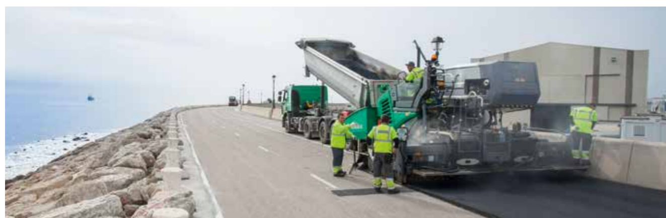
REHABILITATION OF A CAUSEWAY
