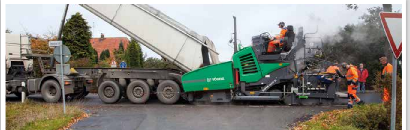
RESURFACING A ROADWAY IN A RESIDENTIAL AREA
