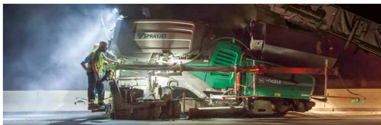
RESURFACING WORK ON A MOTORWAY
