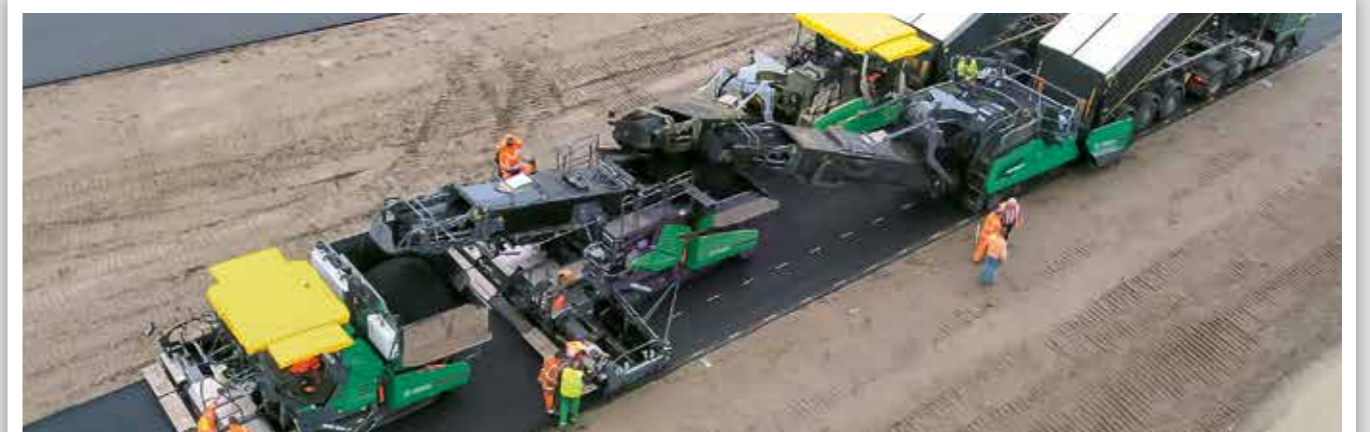
FEEDING PAVERS IN AN INLINE PAVE TRAIN
