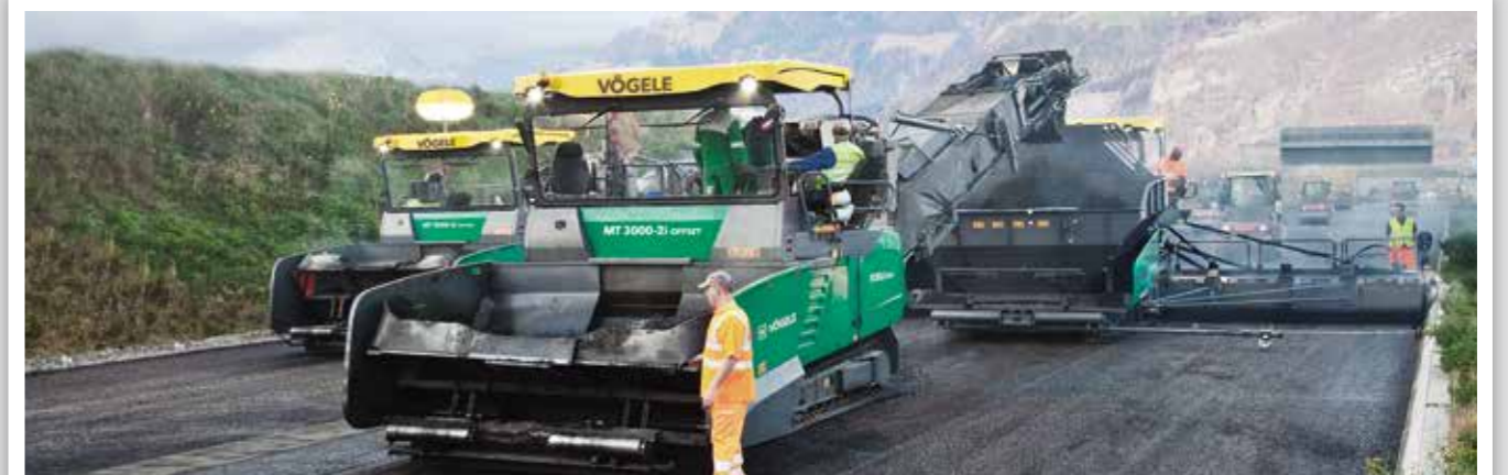
FEEDING PAVERS WHEN WORKING "HOT TO HOT"
